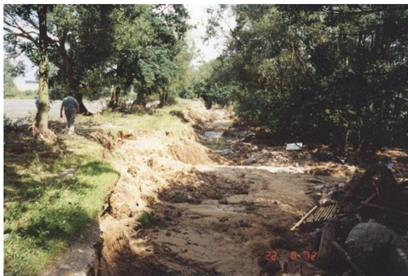
Figure 9. Typical case of the surface erosion during crest overflowing.
