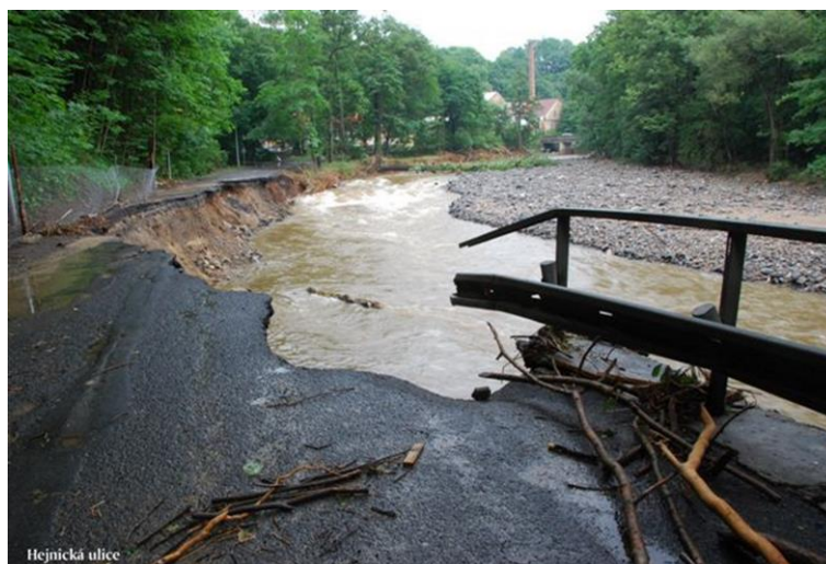
Figure 6. Typical case of damage of road following the water course.
