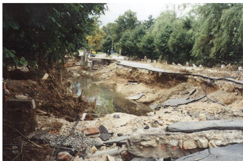
Figure 10. The result of surface erosion of the crest with asphalt pavement.
