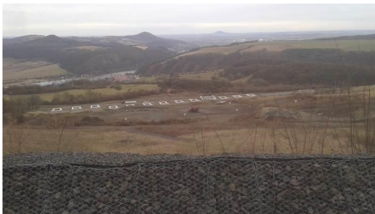
Figure 27. Retaining elements in the lower part of slope.
