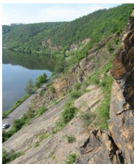
Figure 32. Unfavourable inclination of layers.
