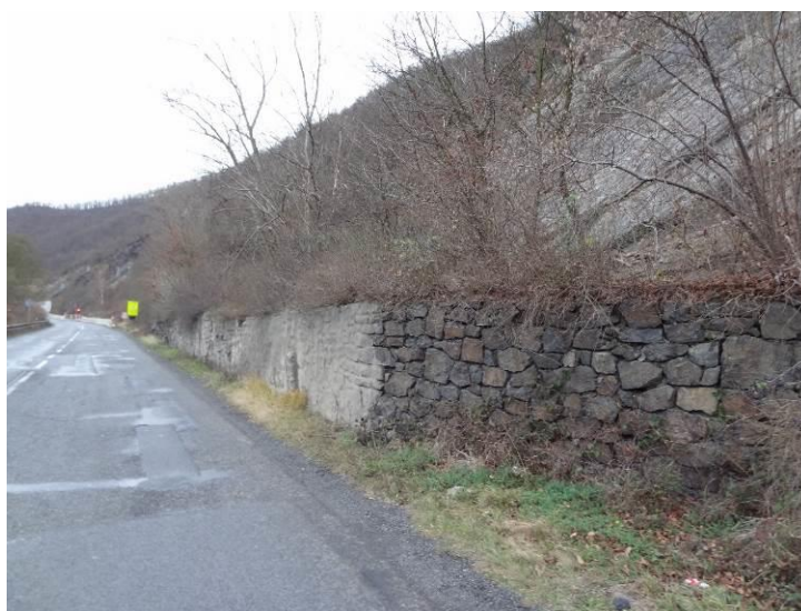
Figure 34. Old masonry retaining wall.
