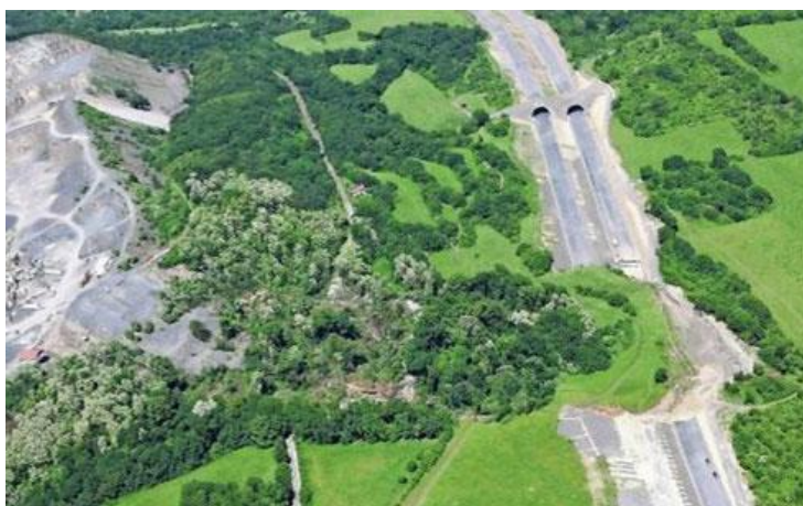
Figure 21. Character of landslide covering the constructed motorway D8.
