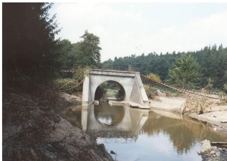
Figure 17. Failed railway embankment on small river Lomnice.
