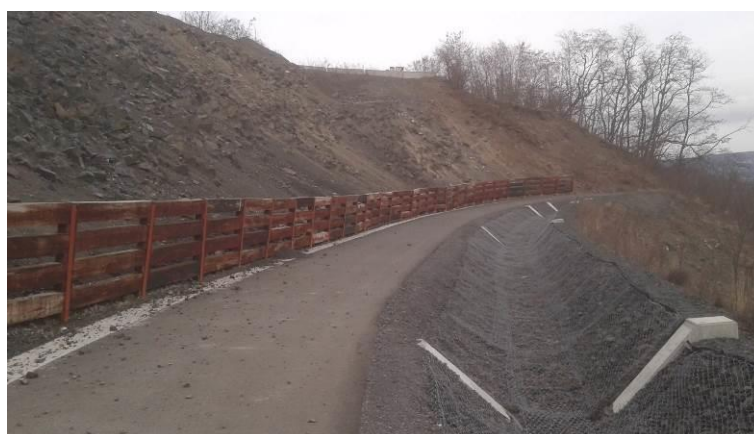
Figure 26. Drainage ditch in upper part of slope.
