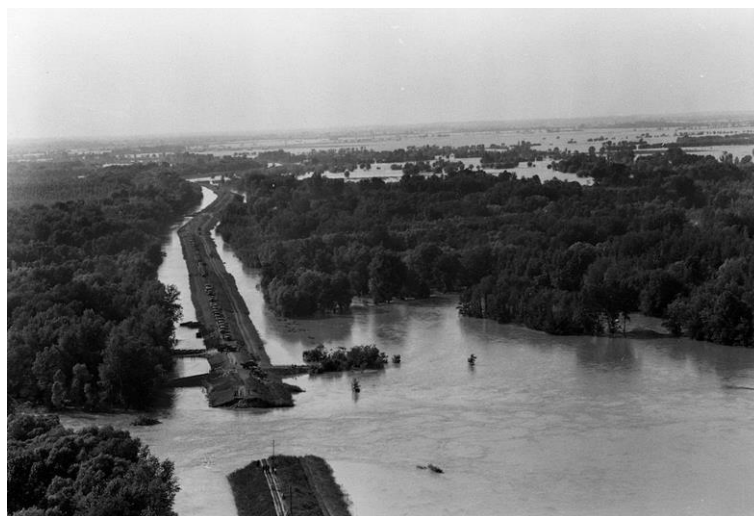
Figure 13. River Danube below Bratislava – example of dike failure, 1965.
