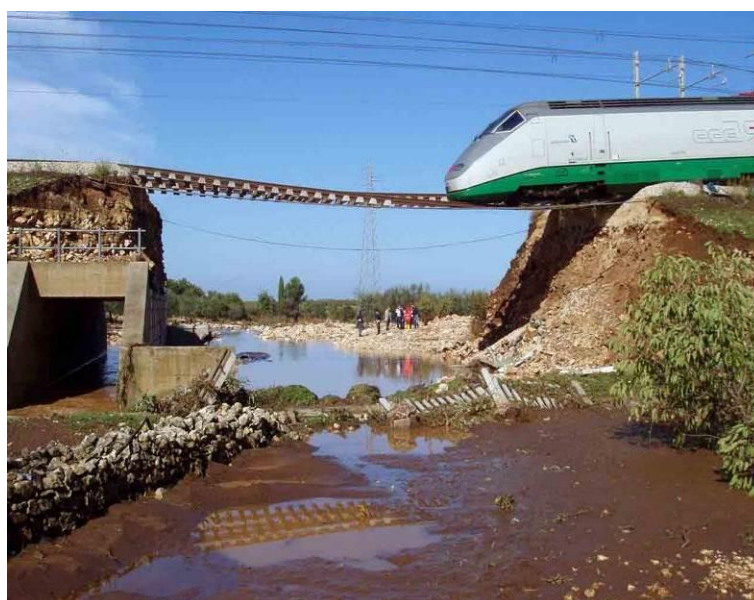
Figure 18. Embankment failure on the railway track Bari – Taranto.
