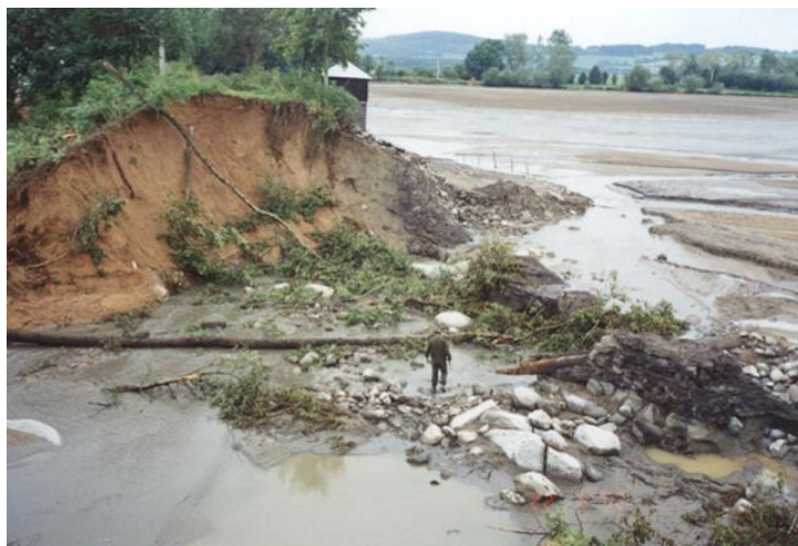
Figure 11. Old timber outlet – the reason of internal erosion.
